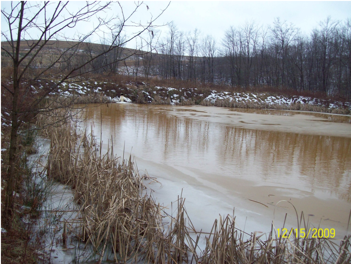
Final treatment pond of the Flight 93 treatment system showing high iron levels
