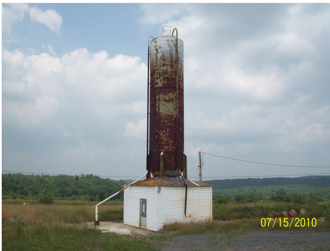
Lime doser, a potential solution for the iron load entering Lamberts Run
